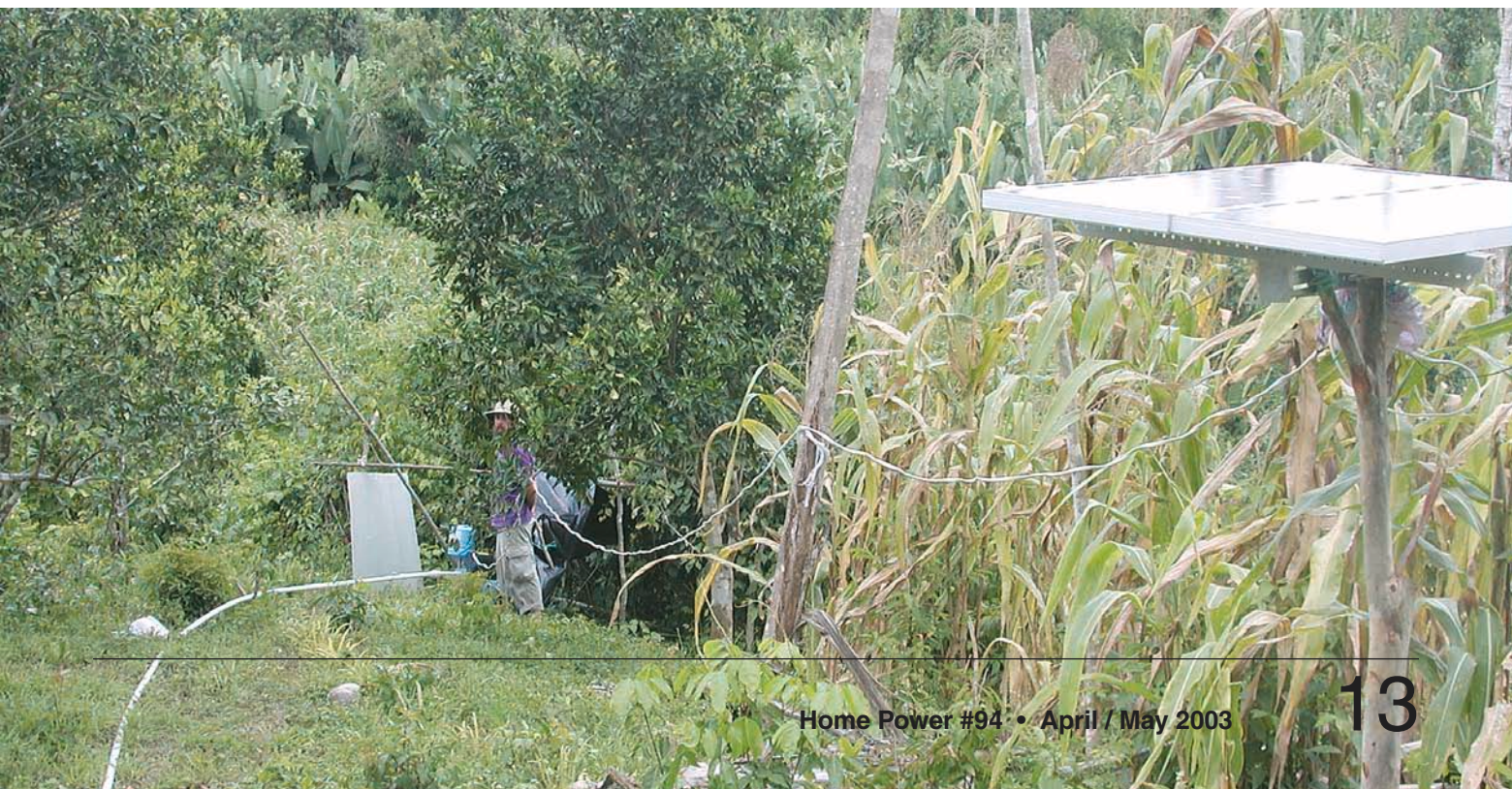
Two BP275 photovoltaic modules directly power the Solar Force piston pumps for two identical pumping systems for organic cacao farmers Ignacio Ash (shown) and Auxibio Sho.
