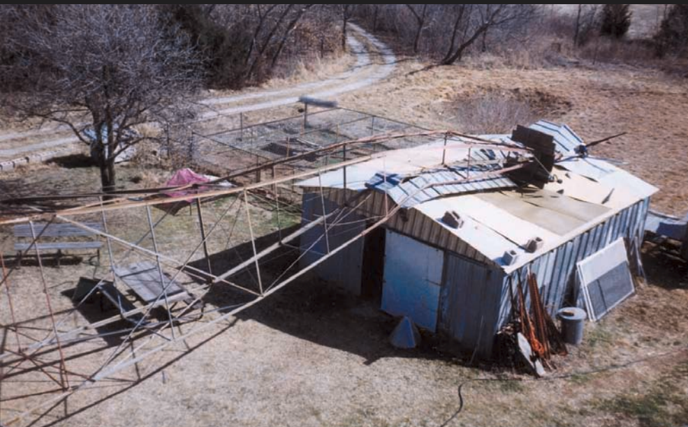
A birds-eye view of the downed tower and smashed shed roof.
