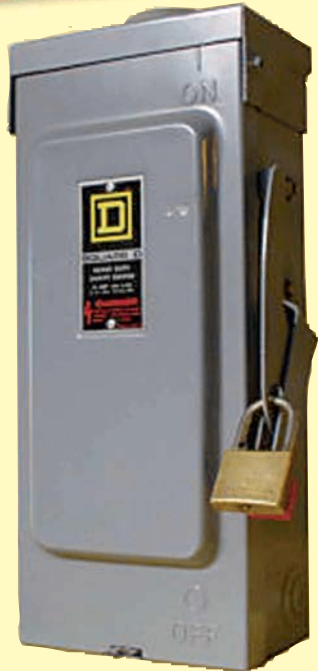
A disconnect in the off position with a padlock to prevent it from being turned on.
