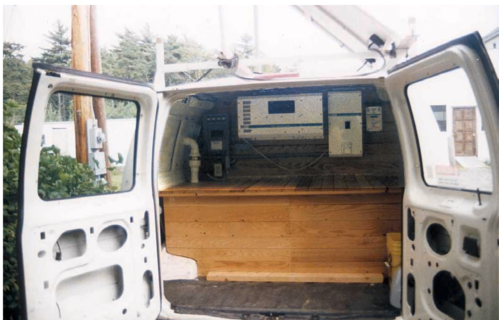
In the back: the battery box and power equipment.
